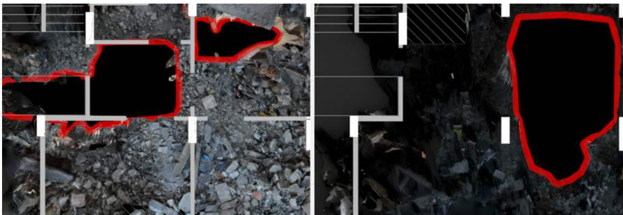
Figure 24: Alignment between perforations to the floor of the TV room and entrance on floor nine (left), and floor eight (right).
