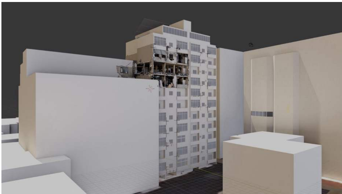
Figure 8: North façade of the Cherri building, showing the site model, photogrammetry model and the sixth-floor window of the neighbouring building (right) where a remnant was found.
