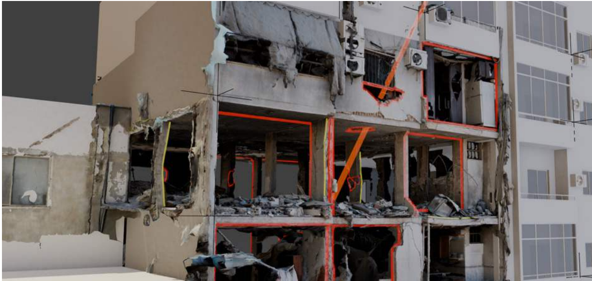
Figure 23: North-east façade view of the alignment between perforations on floors ten and nine, as indicated by the red line.
