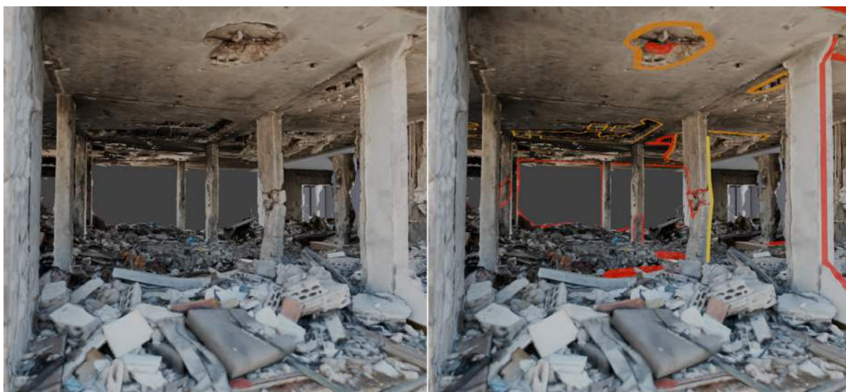
Figure 5: Before (left) and after (right) annotation of perforations (red), surface damage (orange), and distortion (yellow).
