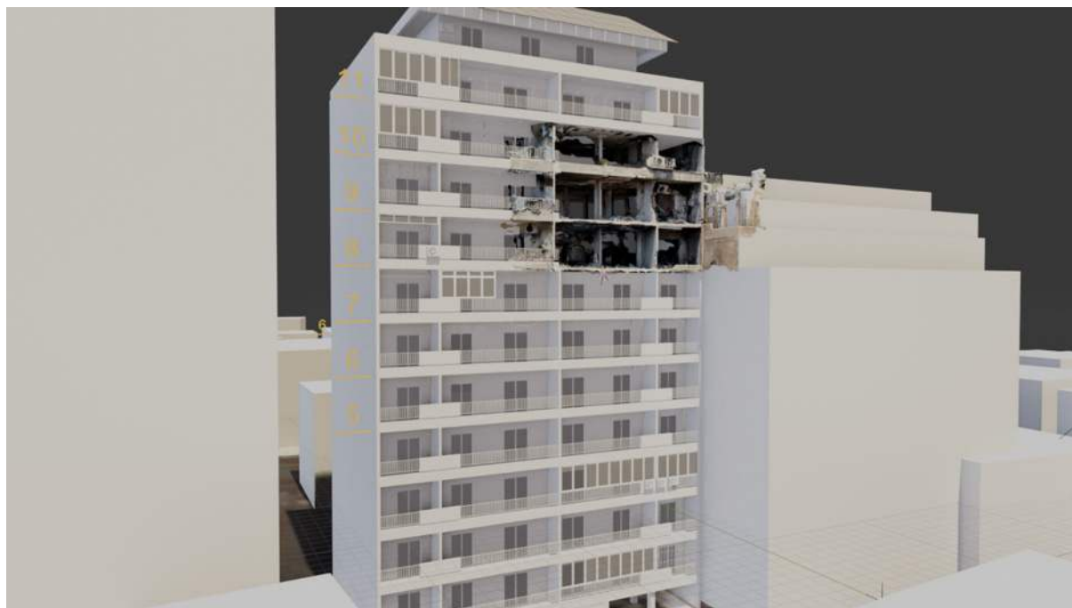
Figure 2: The site model and photogrammetry layer for the south façade of the Cherri building.
