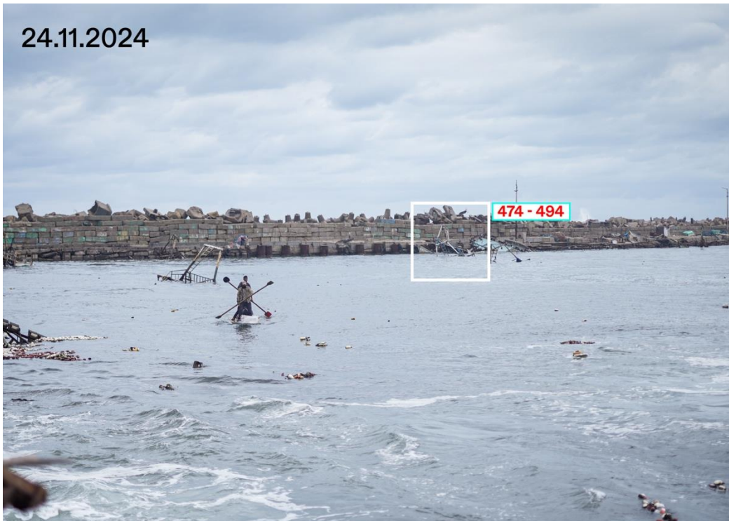
Fig 8. Image documentations of the state of the port on 24 November 2024 by Ain Media Gaza. Annotations by Forensic Architecture mark the location of the boats (in white) and the crater (in yellow).
