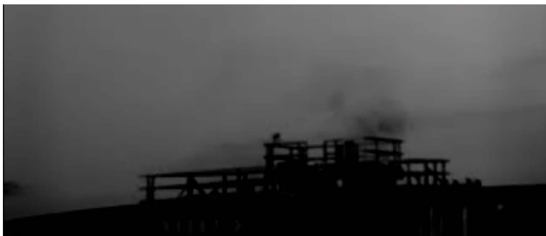
Heated Storage Tank 200-6 was emitting hydrocarbons as documented by Mov0752.
